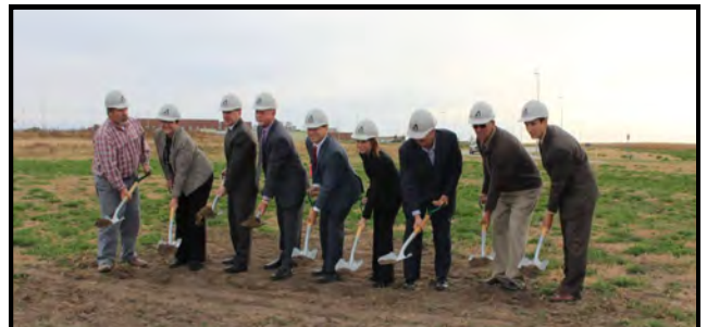
NGage, City and County officials, along with Paul Garnett, Mike Ayars, and Robert Scott took part in the Dialysis Center groundbreaking.
